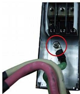
6. Fasten the ring terminals of all remaining wires to the terminal block and tighten each using a torque screwdriver. The appropriate torque settings vary according to the screw size.
